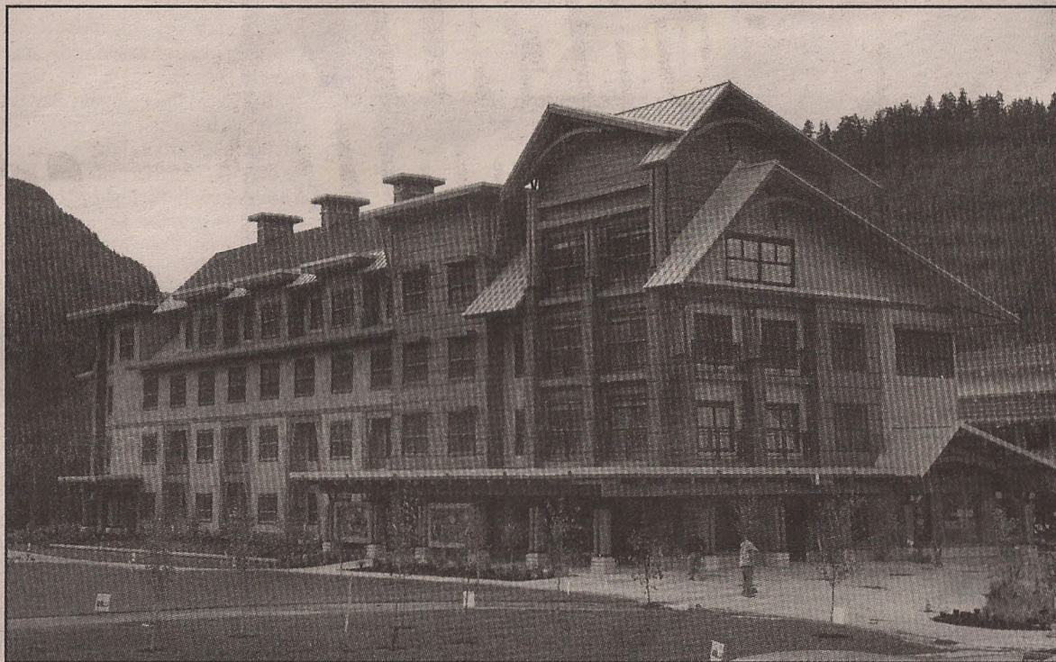
Britco's award-winning athletes' village in Whistler is being converted into affordable housing units.
